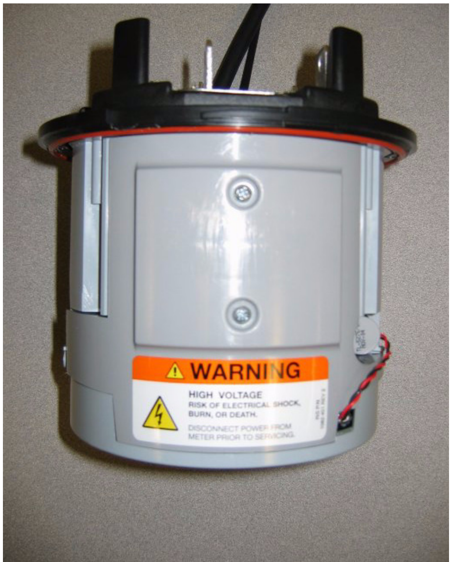
Figure 2.18 Meter with Globe Removed
